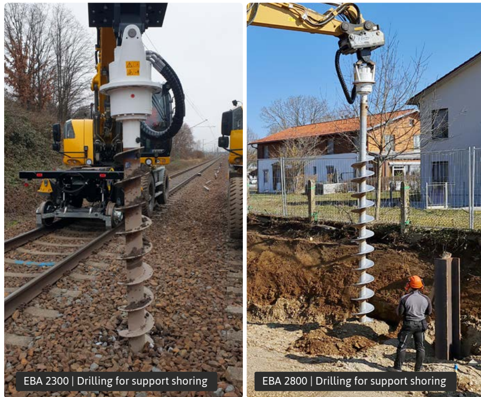
EBA 2300 | Special foundation work
