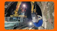
The operator positions the excavator perpendicular to the axis of the tunnel and positions the KEMROC diamond saw on the cable duct at intervals of 150 cm.
