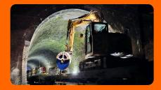
An 8-ton excavator with a KDS 30 diamond saw enters the Elleringhauser Tunnel on a platform truck. The task is to cut concrete cable ducts at the bottom of the tunnel walls.
