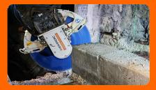
Cutting through the cable duct – with little dust thanks to water spraying. Then the cut section of concrete is lifted loose and loaded for transport.
