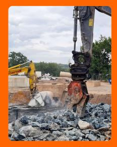
Using the cutter wheel followed by a shearer, the concrete structure was demolished with minimal noise and vibration and, moreover, with high productivity.
