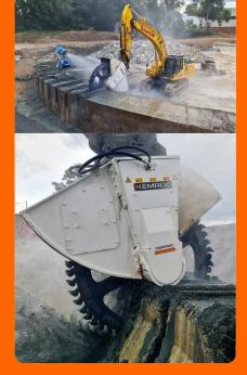
At the Kassel sewage treatment plant, rainwater overflow basins are being replaced. Schnittger cut through the huge, ring-shaped rim of the basin with a KEMROC DMW 220 cutter wheel on a 40-tonne excavator.
