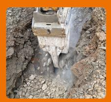
Excavation was quicker with the drum cutter compared to a hammer. The fine-grained milled material can easily be used for backfill.
