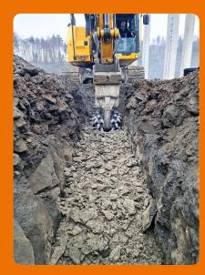
Prior to the construction of a factory and warehouse in Haiger, Germany, Wirth Bau GmbH used a KEMROC EKT 100 milling machine on a 25-tonne excavator to excavate trenches and pits for strip and individual footings.
